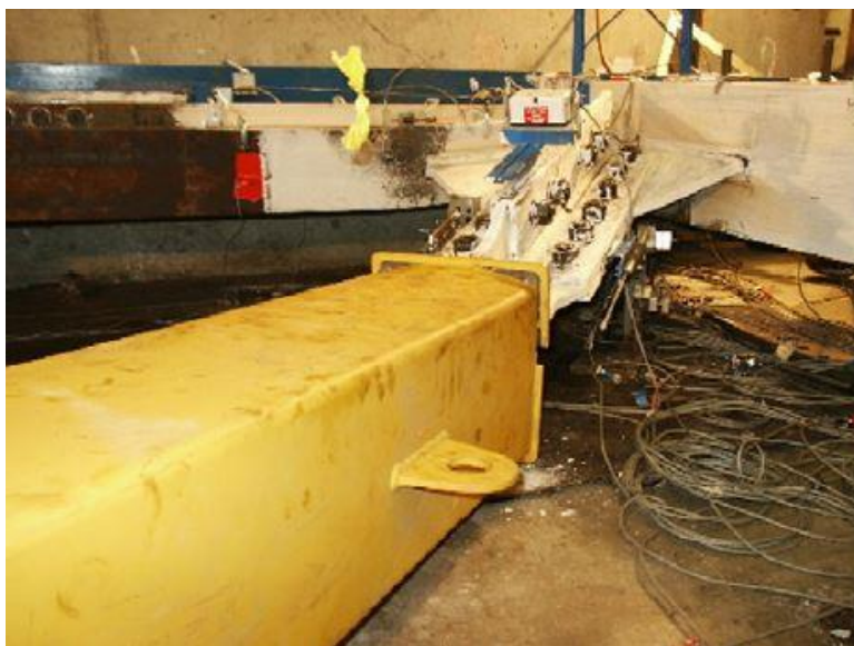
Figure 1.7. Typical connection failure due to out-of-plane end rotation (Palmer et al. 2014)
